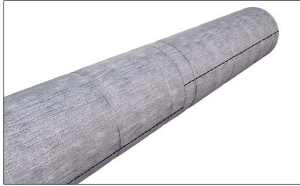
Figure 12: Rotate longitudinal seams to side
