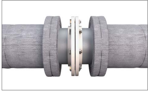
Figure 31: Build up Flange insulation .
