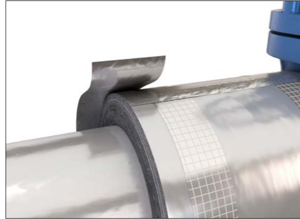
Figure 43: Application of vapour barrier tape at termination
