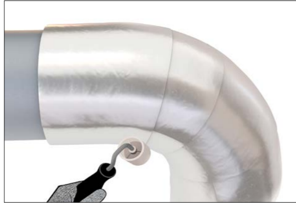
Figure 69: Securing overlaps with roller
