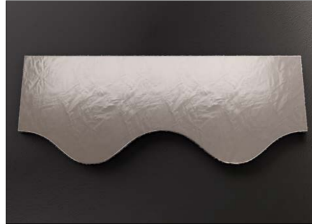
Figure 48: Fabricating the insulation for valve connection
