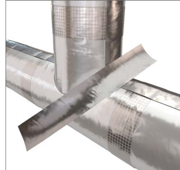
Figure 28: Application of vapour barrier tape
