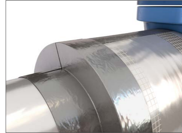
Figure 46: Completely sealed termination
