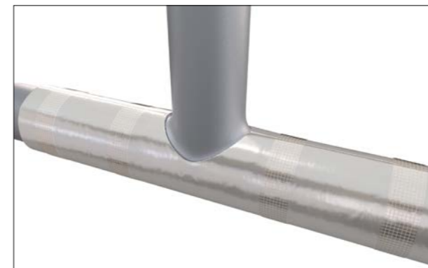
Figure 23: Securing insulation layer with filament tape
