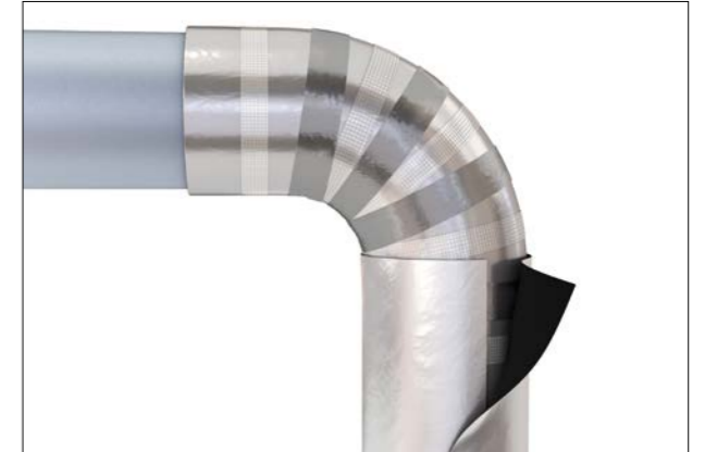
Figure 65: Application of the first bend segment
