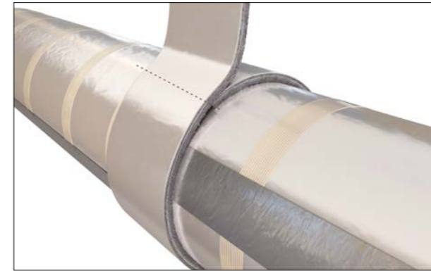
Figure 12: Determining the circumference of insulation for multi-layering
