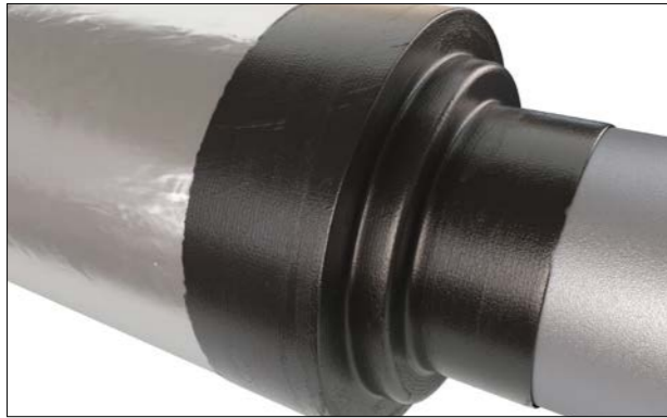
Figure 13: Application of vapour stop at insulation termination
