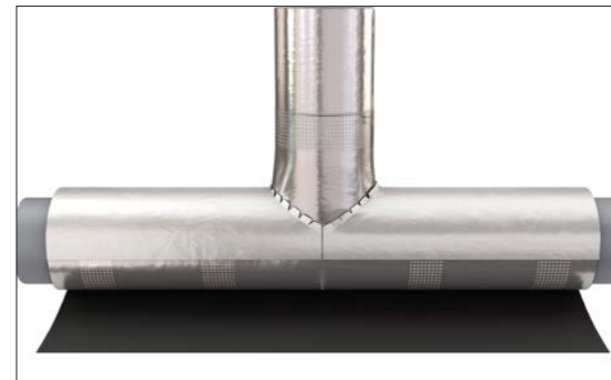
Figure 72: Application of primary vapour barrier on equal tee
