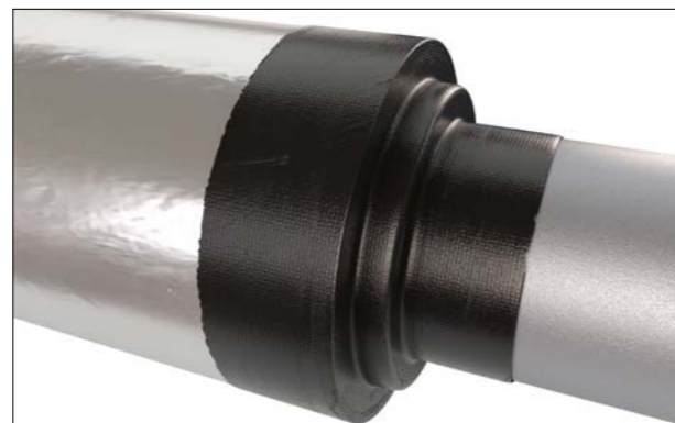
Figure 15: Application of vapour stop
