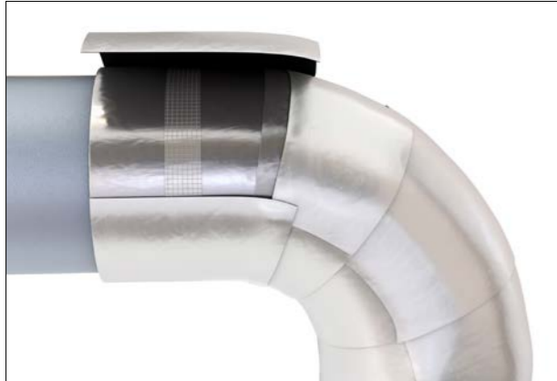
Figure 68: Applying last segment of primary vapour barrier
