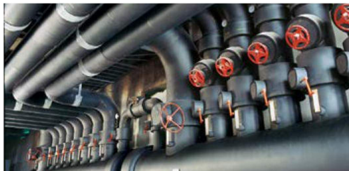
Many advantages described above making Aeroflex suitable for insulating chilled water piping.
