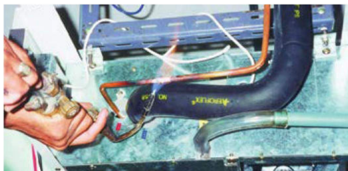
Self-extinguished property, low smoke density, less toxic gases and non-melting characteristic when burnt, making Aeroflex widely used in air-conditioning systems.
