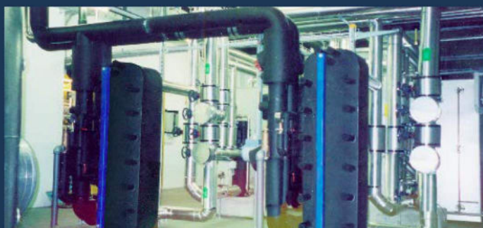
Because of low water absorption and water vapor transmission, Aeroflex is widely used in heating and cooling system.
